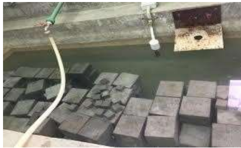
Fig. view of curing
