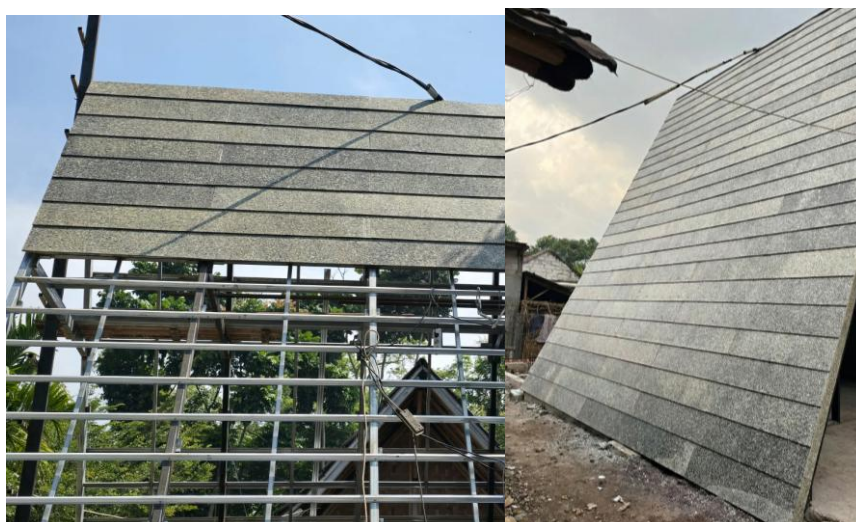
Figure 4. Recycled Plastic Boards for Building Roofs
